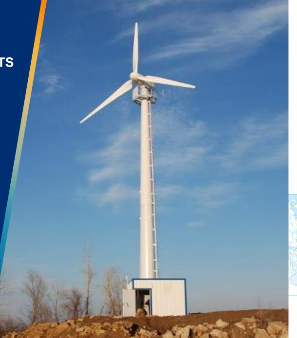
Wind-diesel system with GHRepower 30 kW wind turbine Oil field, Republic of Tatarstan
