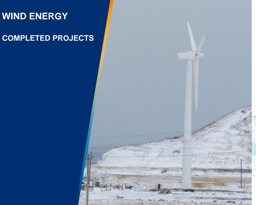
Wind-diesel system with two refurbished 225 kW Vestas wind turbines
