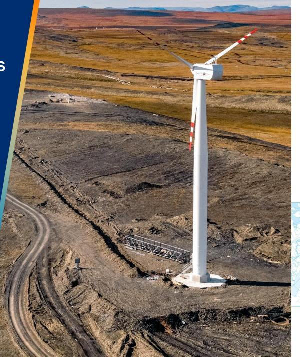
Wind-diesel system with three 300 kW Komai wind turbines
